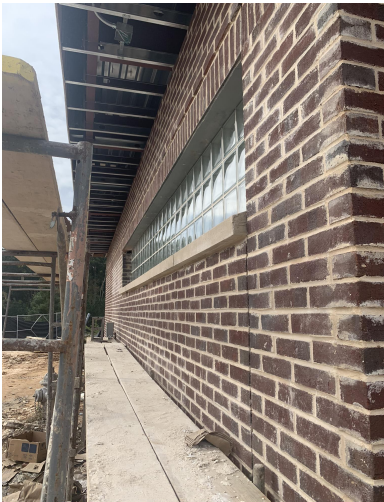
CSK- Glass Block Install
