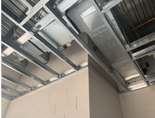
CSK- Duct Work Install
